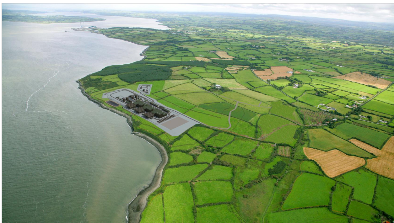
Figure 2.2: Site of the Proposed Development (Aerial)
